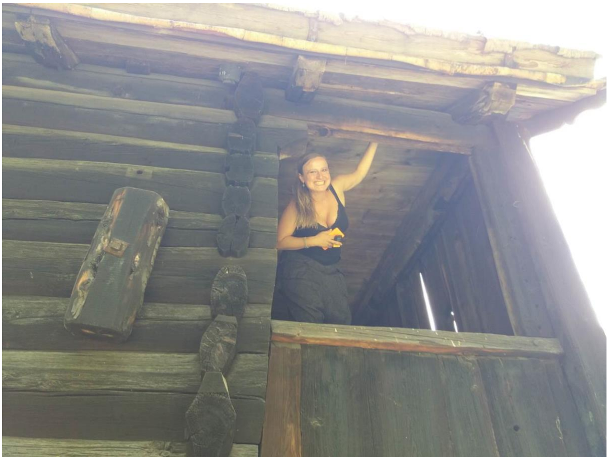
Figure 11: Transformative Envelope on the Loft from Raundal, Voss 1600–1700 – Oslo Open Air Museum. The envelope of svalgang (on the right) can be fully or partly removed or fully be closed again (photo: Raková 2017).
