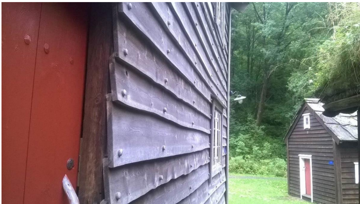
Figure 12: Responsive Wood Envelope of Loft from Dale, Fusa 1700 – Hordaland Museum. The envelopes here have the left side of the plank oriented towards the inside and are attached on the lower side of the panel. Thus in dry weather the plank warps towards the interior and in wet weather generates enclosure together with the upper panel (photo: Davidová 2017).
