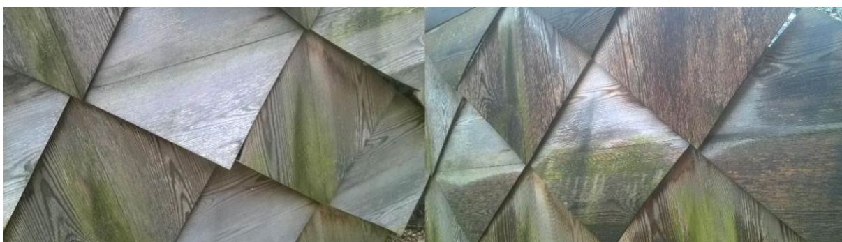
Figure 23. Ray 2 Responsive Wood Envelope Prototype: a) in semi-dry April weather when the screen is partly open for a boundary exchange between the exterior and the semi interior; b) After a light rain in April when the System is closed to prevent the humid and cold air from passing through the boundary; both after four years of exposure to weather and biotic conditions. The prototype became inhabited by Blue Stein Fungi, Algae and Lichen. These, especially the algae, regulate the moisture content of the wood, thus contributing to its warping. Notice also the organisation of the Algae habitation caused by the material's fibre direction and position within the design, which is affected by material performance and form. Thus, it is organised through its moisture and the organisms' abundance and distribution interaction (photo: Davidová 2017) (Davidová, 2017a).
