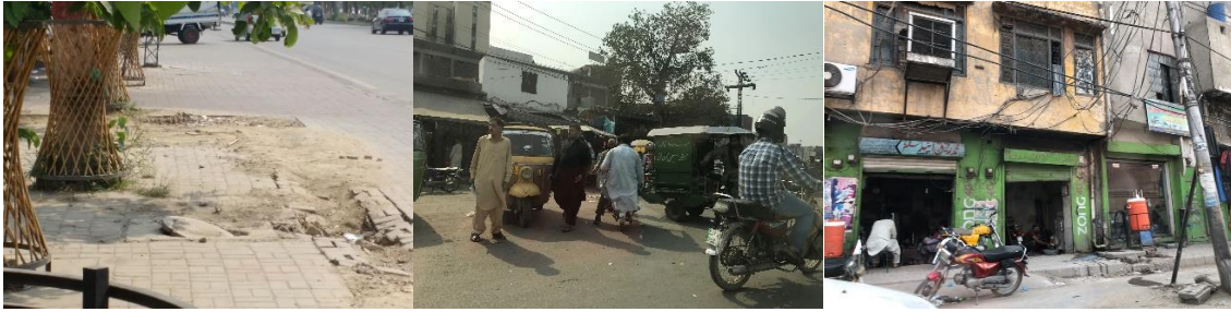
FIGURE 2. Poorly maintained pedestrian areas in Lahore (Photograph: WEMOBILE project, 2018)
