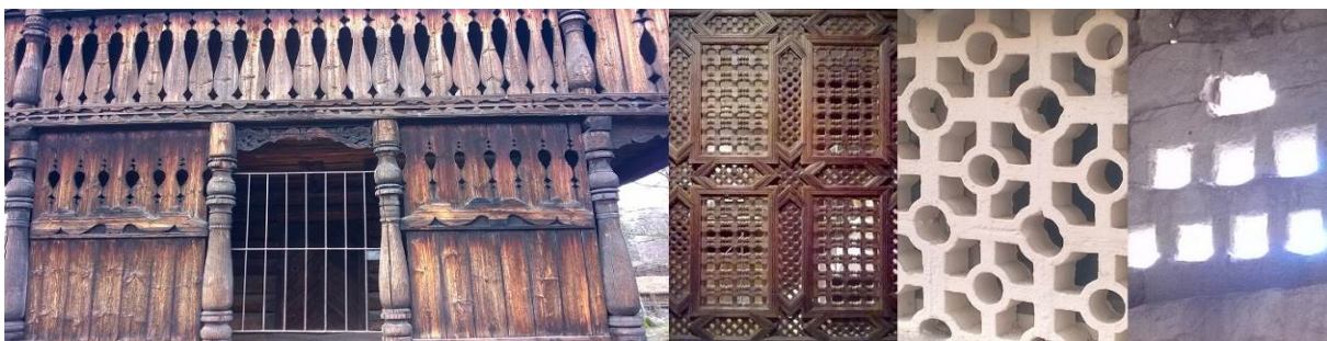
Figure 11: 'Breathing Walls' in vernacular architecture: from left to right, a) Norwegian svalgang (a semi-interior space) screen of a habitable loft from 1797, Oslo Open Air Museum, Norway (Photo: Davidová, 2016); b) Moroccan mashrabīya separating different climatic and privacy layers of the onion principle of a traditional Turkish house from about the 15th century, Houston Museum of Fine Art, USA (Photo: Davidová, 2016); c) traditional south Portugal screen wall in Fishermen's Village, Salema, generating a semi-interior micro-climate between a street, a courtyard and a house, Portugal (Photo: Davidová, 2016); d) Çavuşin Monastery's human-pigeon house from 964/5, Cappadocia, Turkey (Photo: Davidová, 2016).
