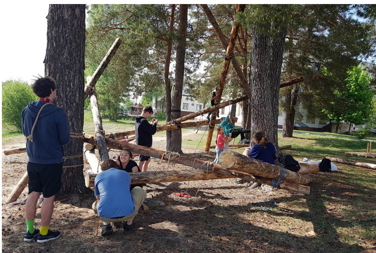
Figure 18: The construction site of the Co-oCo-oNest prototypical semi-urban intervention (Photo: Davidová, 2018).
