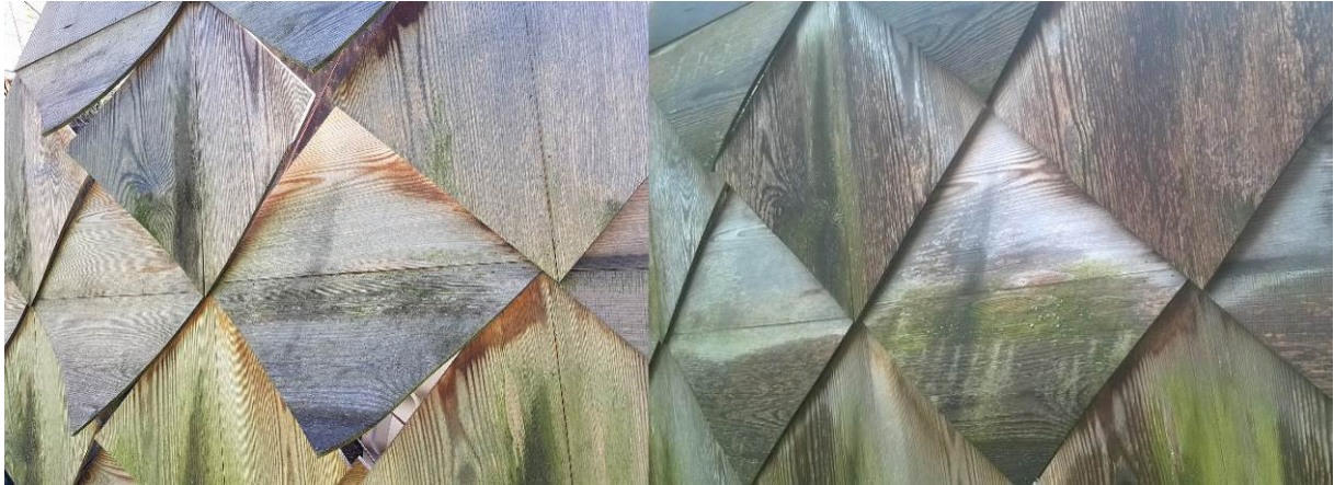
Figure 7: Ray 2*2013 Responsive Wood Envelope Prototype: a) in semi-dry June 2018 weather when the screen is open for boundary exchanges between exterior and semi-interior; b) after light rain in April 2017 when the system is closed, which does not allow the humid and cold air to pass through the boundary after five and four years, respectively, of exposure to weather and biotic conditions (Photos: Davidová, 2017 - 2018).
