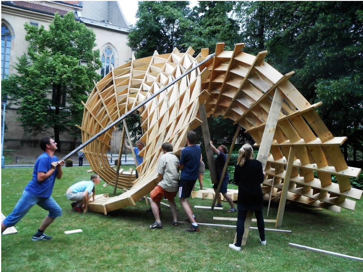
FIGURE 6: Erecting of the Loop pavilion at site 1 (photo: Davidová, 2014).
