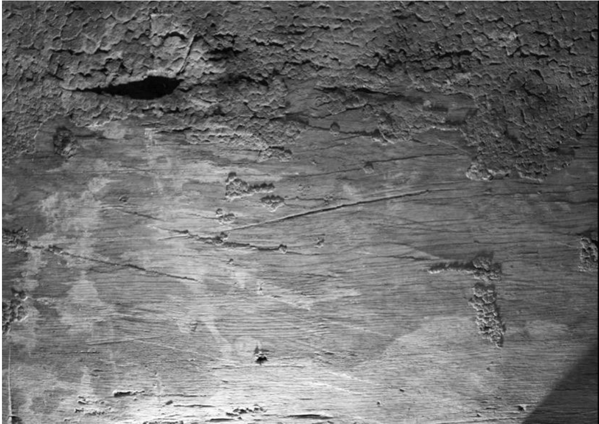
FIGURE 8. Traces on the wall-plate eventually from an adze similar to 21592:63 in the Mästermyr find.
