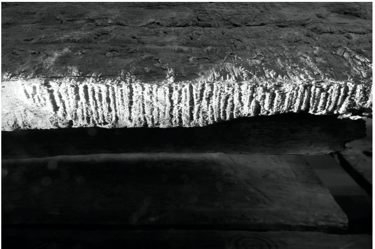
FIGURE 10. Traces from a saw-blade on the side edge of the wall stave SHM 10232:43.
