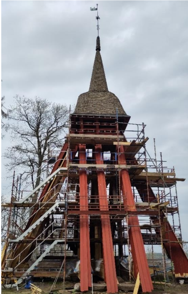
FIGURE 2. The belfry of Kungslena church in Skaraborg, Sweden, was built in 1679 and renovated several times, most recently in 2023. During this last renovation, most of the cladding of the lower half was replaced, whereas the higher part, protected by the roof, has probably been standing for hundreds of years and is still preserved today.
