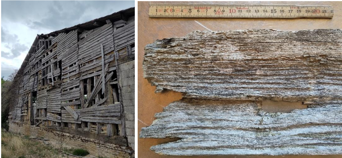
FIGURES 9 AND 10. The West façade of a house built with timber-framing and wattle and daub filling in Frampas, Champagne, France (Figure 9). The façade was covered with uncoated tavillons made of Alder, many of which came off, leaving the filling unprotected and washed out by the rain. A sample from this façade is showing a nail hole, which has become bigger and where crack formed from it to the edge of the tavillon (Figure 10). The abrasion of wood around the nail is mainly due to small movements between wood and metal combined with erosion. It is obvious here that widening of nail holes eventually makes cladding non-functional as a protective layer.
