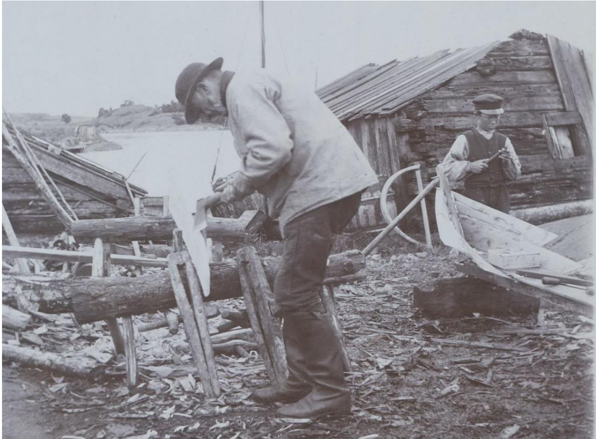
FIGURE 1. Boatbuilder building an öka in Stockholm Archipelago in the late 19th century. Photo by Axel Sjöberg.
