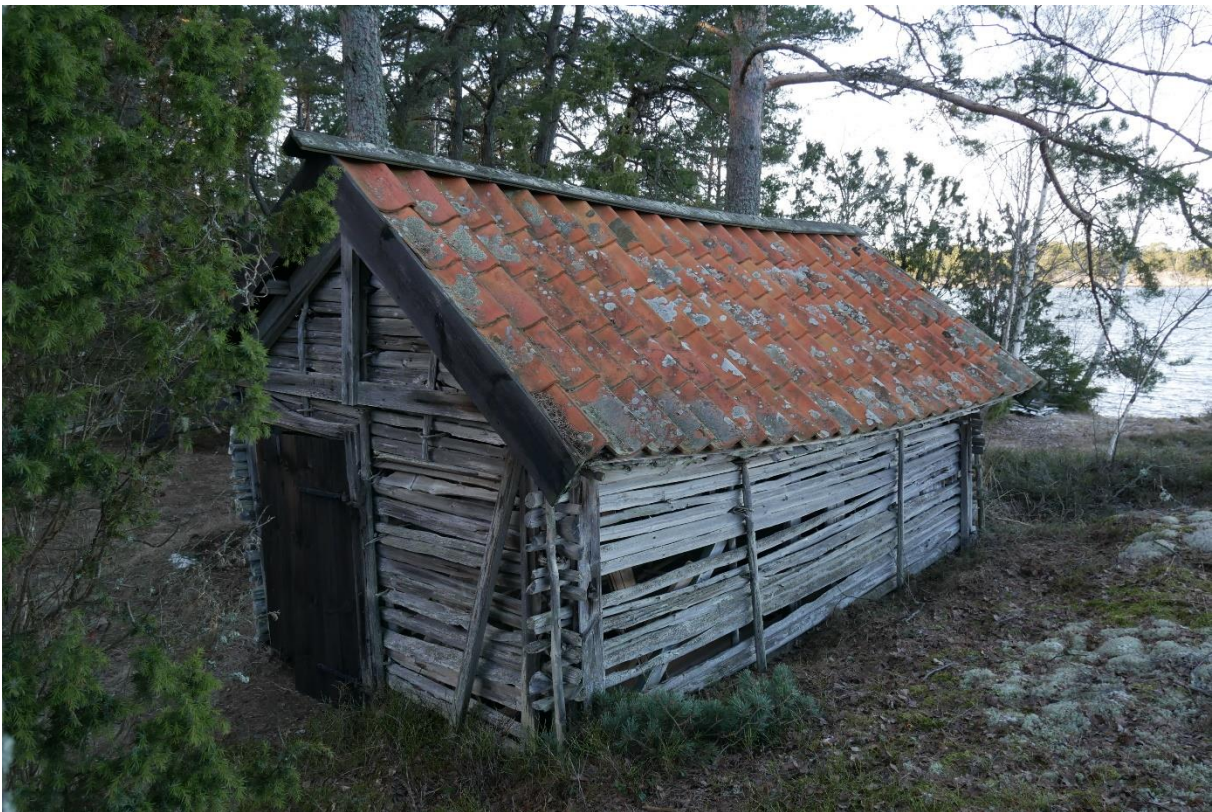
FIGURE 3. One of the few still standing wooden pole fence buildings; Pelle Duvas boat shed in the province of Södermanland, Sweden, built in the 1890s (Svantesson, 2023).
