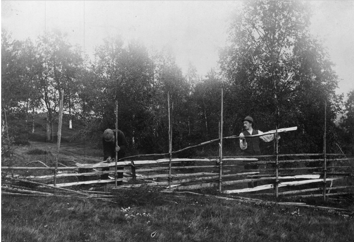
FIGURE 1. Construction of a wooden pole fence in the 1920s, province of Värmland, Sweden (Keyland, n.d.)
