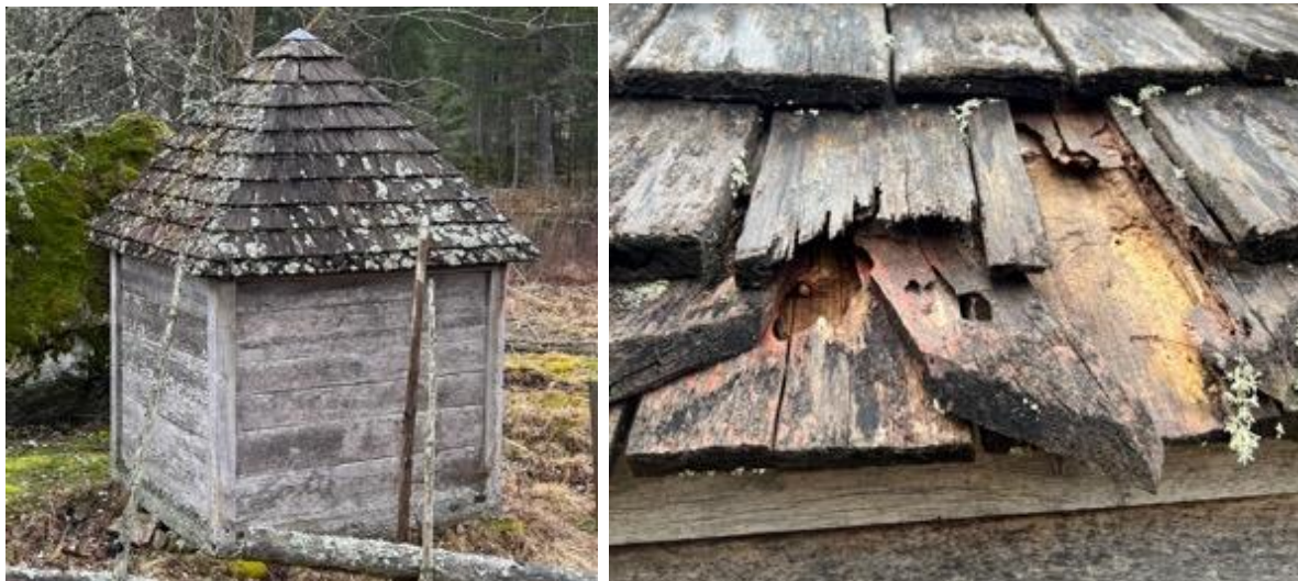
FIGURE 8 AND 9. To the left: The aspen roof is still in good condition even though it is shaded by vegetation. A few of the shingles have deteriorated. To the right: As in Tönnersjö, the shingles have a soft surface that can be peeled off. However, we saw no insect holes. Börje used aspen trees with few branches and a diameter of about 25 cm. The shiny silvery grey surface was obvious and reminded of photos of Russian aspen roofs from the Kizhi outdoor museum and roofs on churches in Åland.
