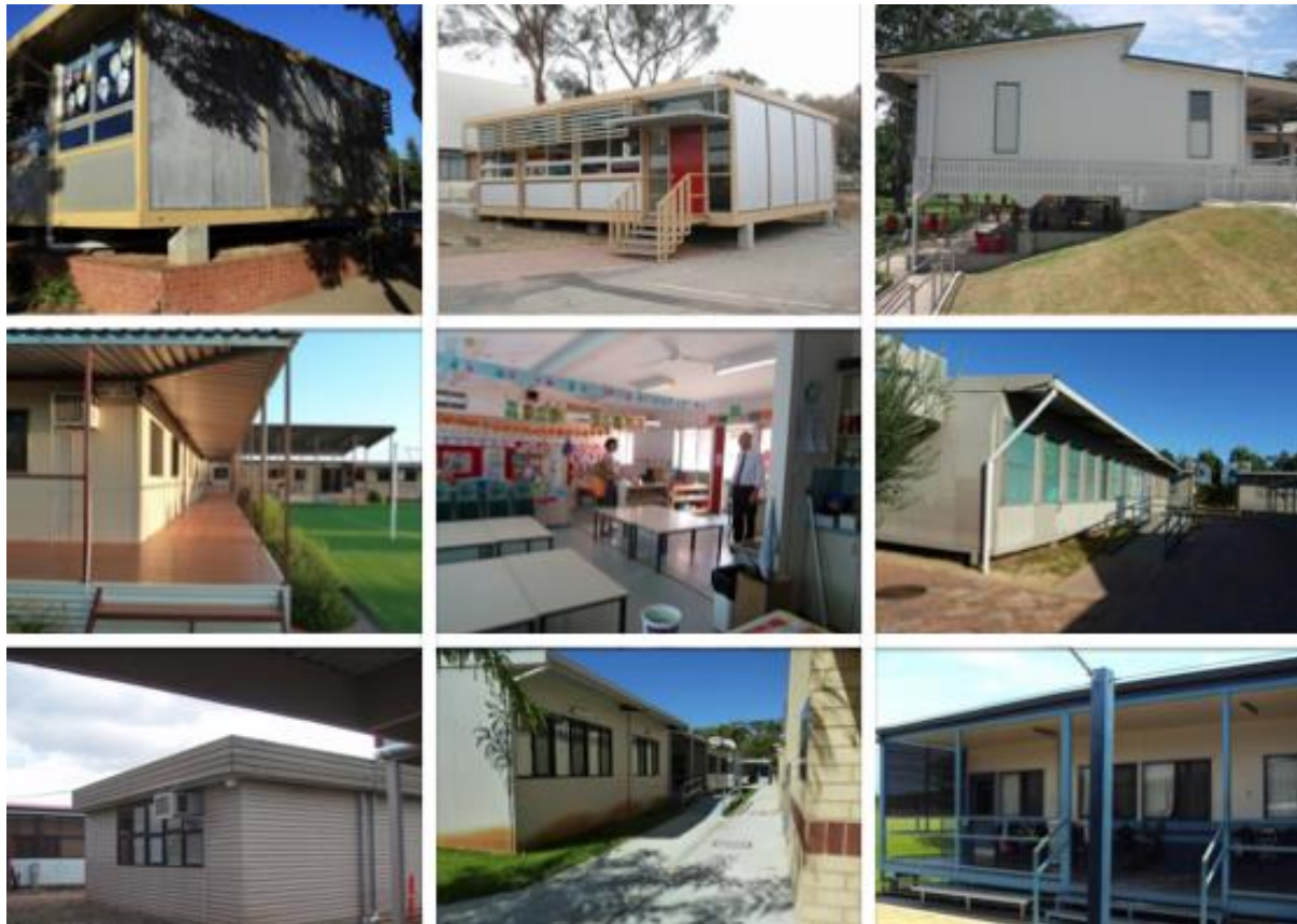
Figure 2: Examples of relocatable classrooms across Australia (Source - FPS Research Team)
