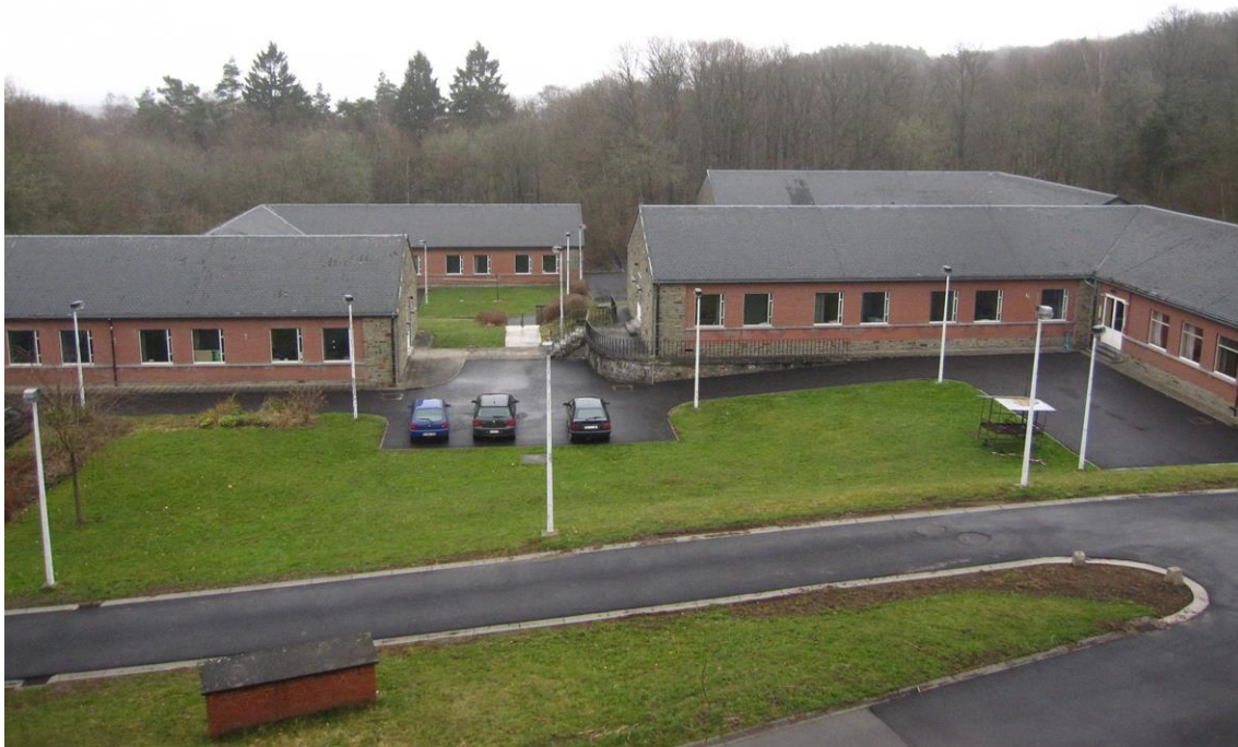
Figure 4. Existing dormitories, to be demolished and replaced.
